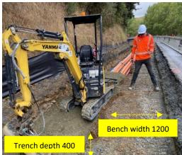
Photos from the incident scene: Left – Excavator toppled over; Right – Trench dimensions;
