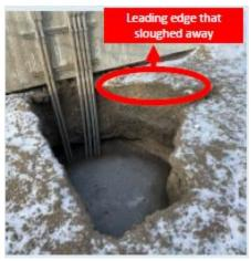
Opened hole after hydrovac operation  $1m \times 1.5m \times 1.5m$
